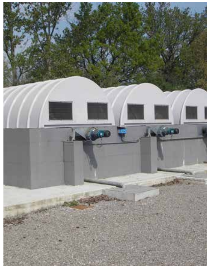
Concrete tank installation San Rigo (RE), Italy
